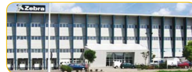
Heerenveen site, the Netherlands
